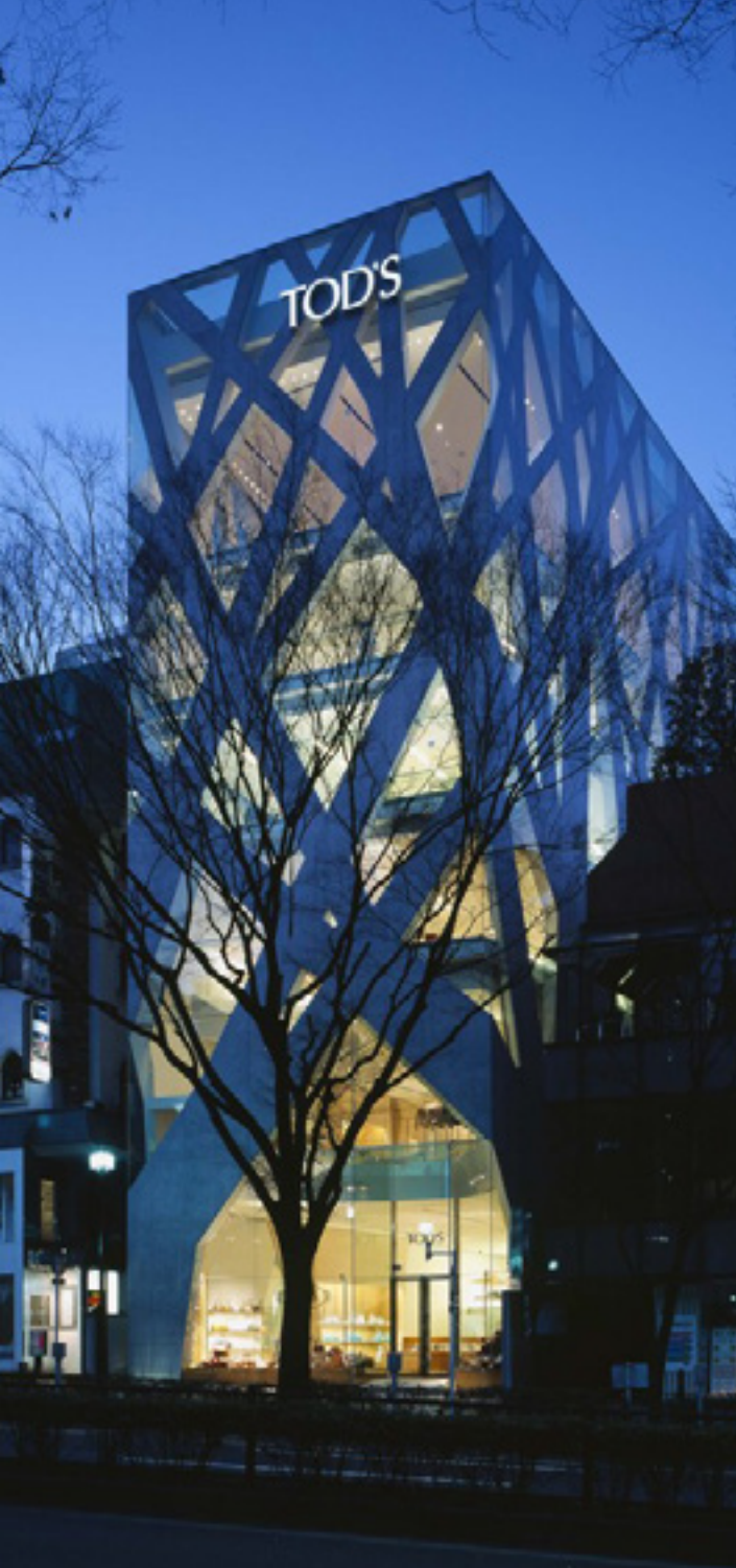
Tod's designed by Toyo Ito
