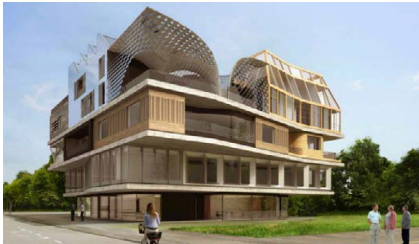
Modular "plug and play" building to test sustainable systems, materials, and technologies. "NEST will be a dynamic demonstration platform where researchers can insert and test various components building modules." Source: http://inhabitat.com/switzerlands-nest-high-rise-is-a-modular-test-bed-for-the-future-of-green-building-technology/
