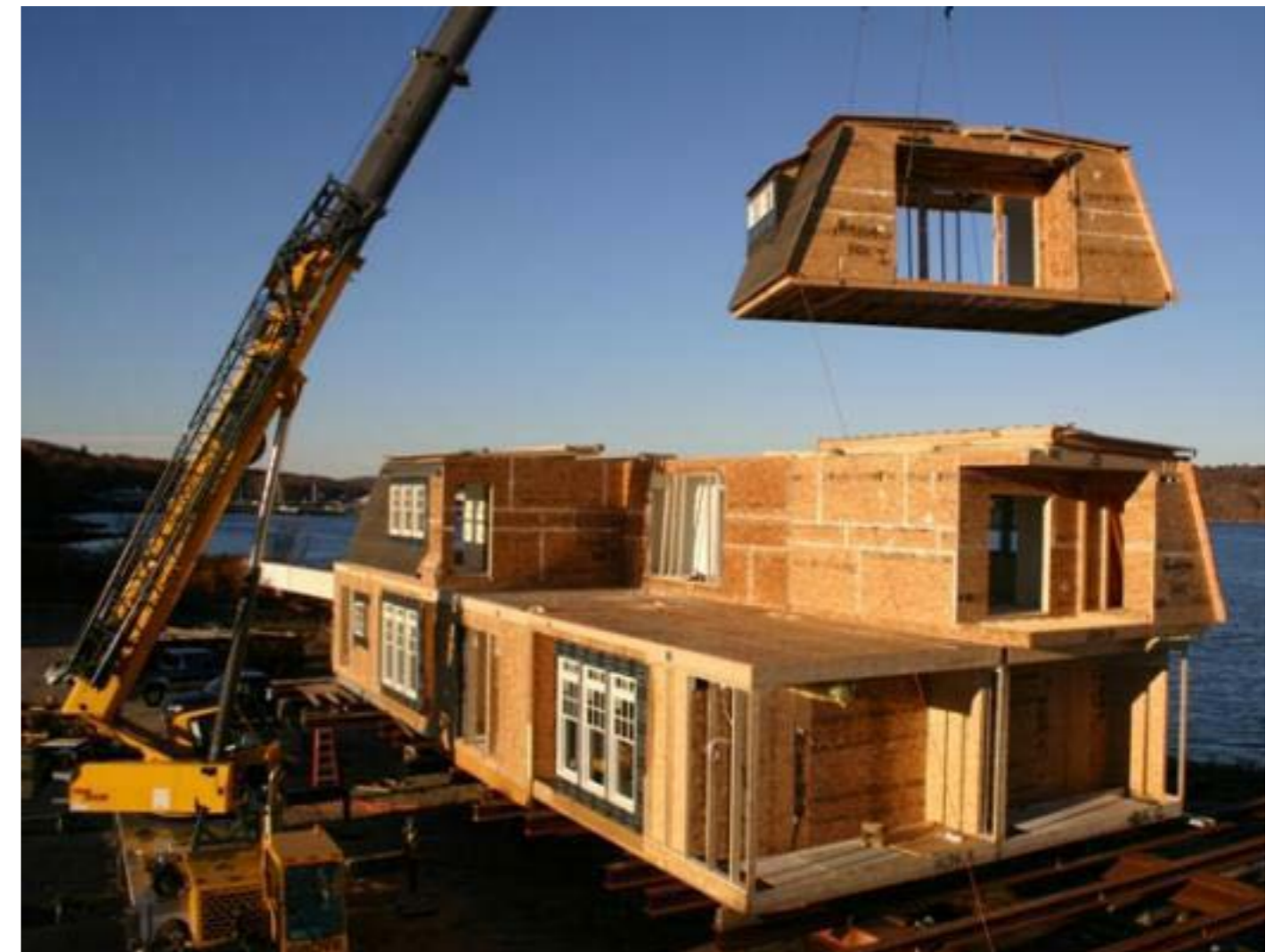
Modular construction of a timber house Source: http://raconteur.net/business/top-ten-construction-innovations
